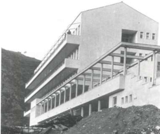
Fig. 8 Health Center Risan, (Source: Blagojević, 2003: 95)
