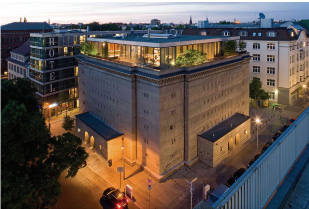
Illustration 4. Boros Bunker Berlin. Built 1942 as air raid shelter for 2,000 people in the “classical” style.
